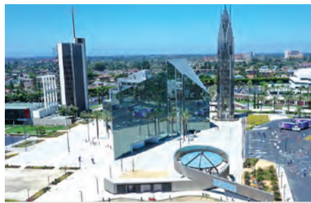
Project: Our Lady of La Vang Nominee(s): Gray West Construction Inc. Anna Zhang, Senior Project Manager John Thome, Vice President, A&E / Preconstruction Tim Butz, Site Manager Eric Clara, Estimator Paul Buster, Superintendent
