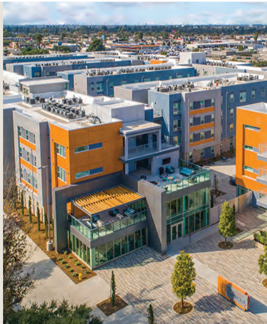
Project: The Harbour at Orange Coast College Nominee(s): Servitas Angel Rivera, Senior VP of Development Services HPI Architecture Ammar Sarsam, Principal Michaela McClelland, Senior Associate Moss & Associates Dale Rowton, Superintendent Shane Arnold, Project Manager MHP, Inc. Structural Engineers Rick Beall, Principal James Kramer, Associate Principal Design West Engineering Jonathan Bianchet, Project Manager
