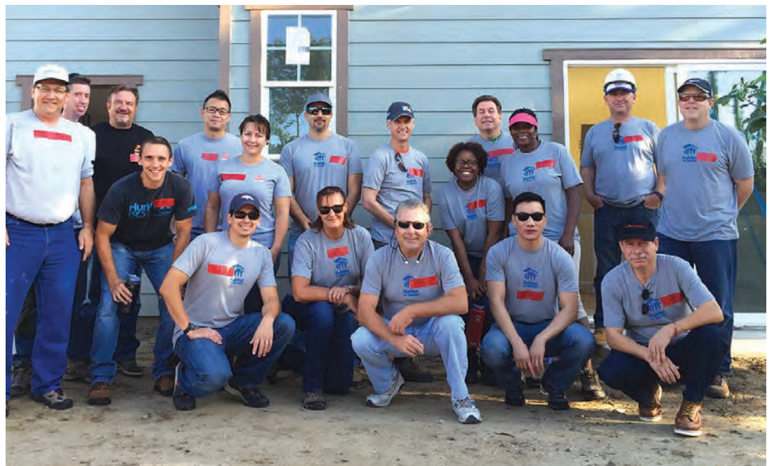
Fluidmaster, Inc. employees traded their smartphones for hammers during a Team Build Day where they helped build affordable Habitat for Humanity of Orange County homes.
