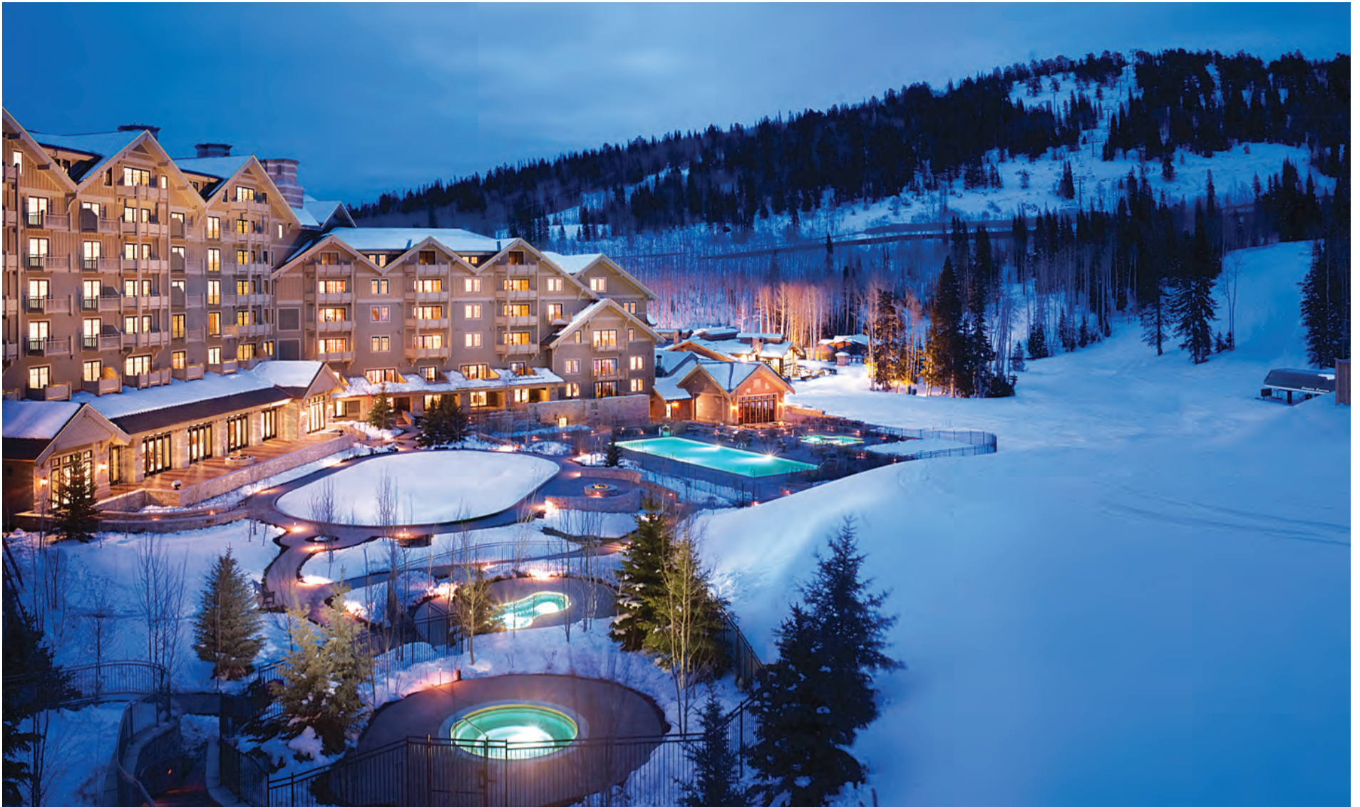
Montage Deer Valley, Deer Valley, Utah, Built by Layton Construction, 2010
