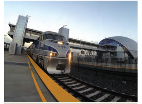
Project: Anaheim Regional Transportation Intermodal Center (ARTIC) Nominee(s): Clark Construction Group – CA, LP Dave Burrus Parsons Brinkerhoff Samuel Sims
